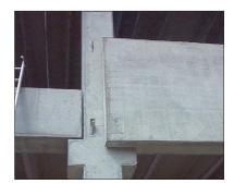
One of two precast cladding panels, shown at the SureClad Lock locations, has been positioned, leveled and attached.
