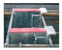
Two SureClad Locks, shown with the locks retracted behind cover plates, are positioned and reinforced in a precast form prior to concrete placement.
