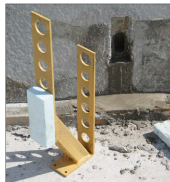
After the installation is complete, there is only a very small opening to patch.
