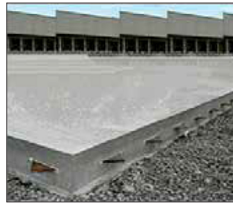
Dowels are inserted into sleeves after edge forms have been removed.
