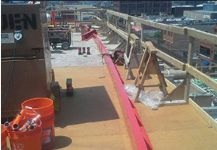
Numbered Slab Edge Forms make it easier to repeat the floor plan on every story, every time.
