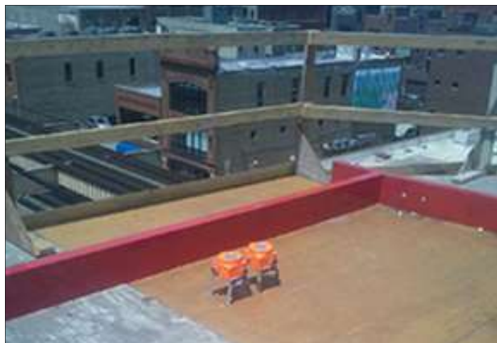
Ends can be overlapped or Slab Edge Corners and Fillers can be supplied to match the floor plan.
