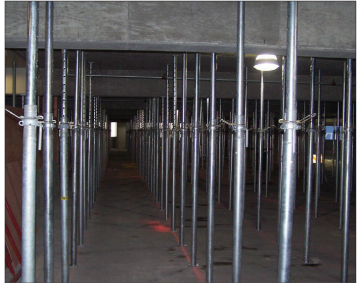
Post Shores can be used for supporting plywood decks or reshoring existing structures.
