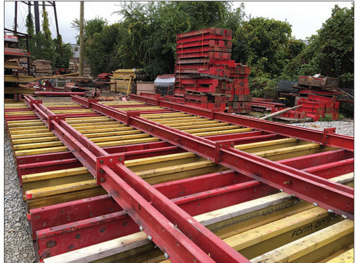
Butt Plate Walers, bolted together end-to-end, are used to support this large wood beam gang.
