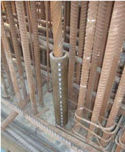
Repair and Retrofitting
