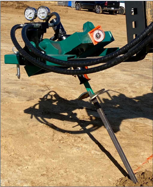
A skidsteer with a torque motor attachment is used to install the Helical Ground Anchor at the prescribed angle and depth for bracing.
