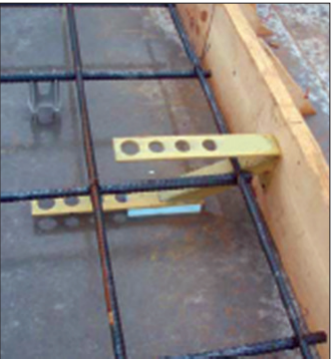
The Slant Anchor is simply positioned and nailed to the form.
