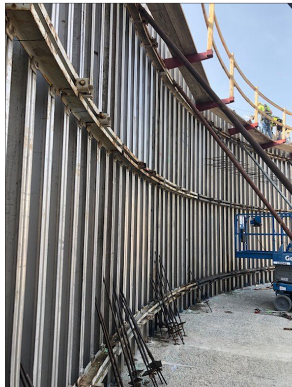
Radius forms can be reconfigured to match changing radius and wall dimensions.
