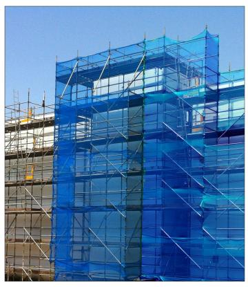
SureNet mesh enclosures are an easy way to separate construction activities from surrounding spaces. SureNet mesh can reduce the risk of falling materials, fasteners, tools and debris.
