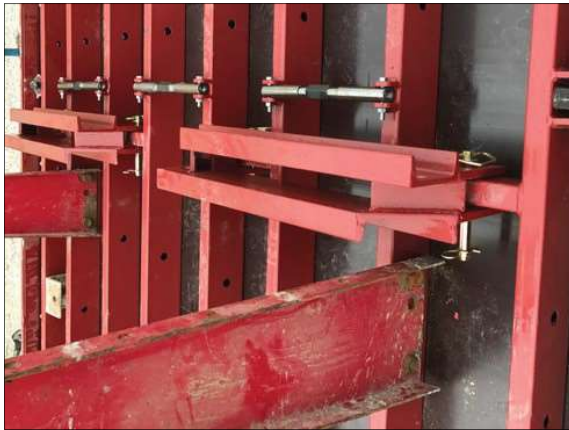
Walkway brackets bolt to panels to provide support for work platforms.
