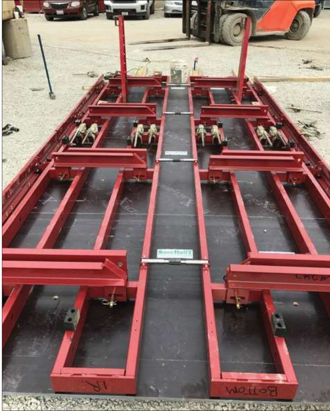
The SureCurve panels can be assembled into a gang, including all the connecting hardware and accessories, while safely on the ground.
