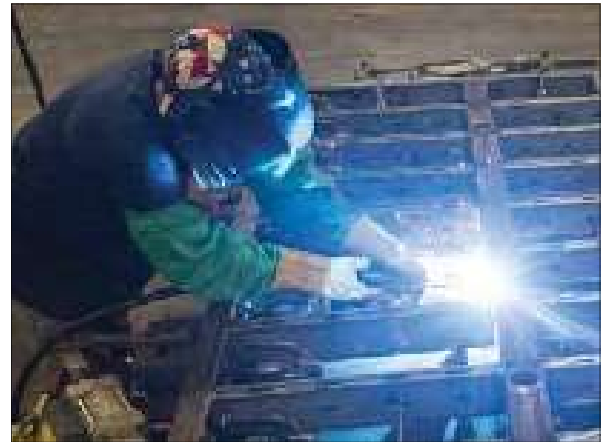
Precision welding turns components into a single structural frame.
