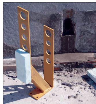
After the installation is complete, there is only a small opening to patch.
