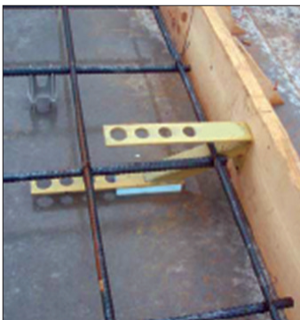
The Slant Anchor is simply positioned and nailed to the form.
