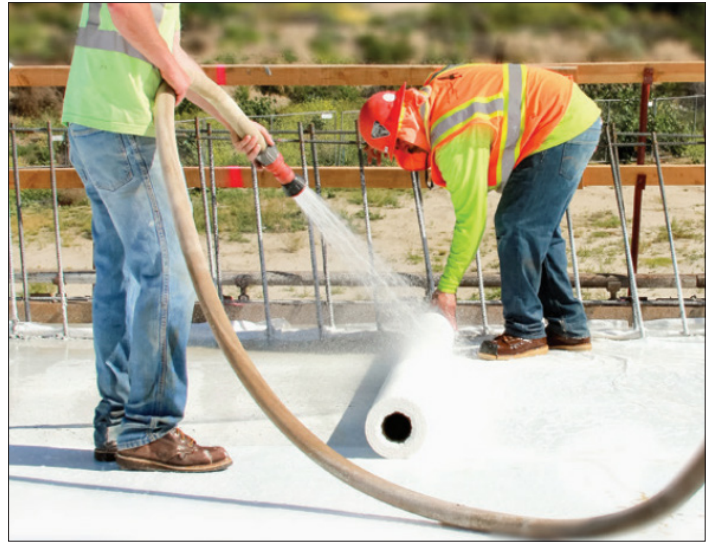
Vertical & Bridge Concrete Curing Blanket
