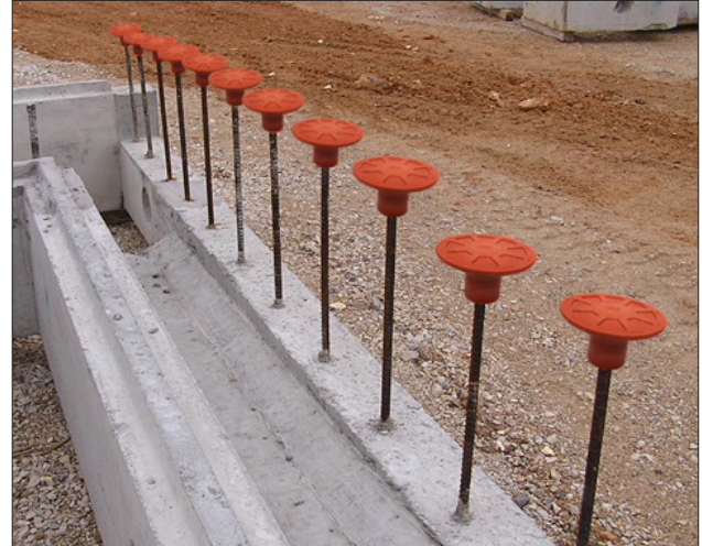
Prevent injury and impalement on work sites with orange Rebar Safety Caps.
