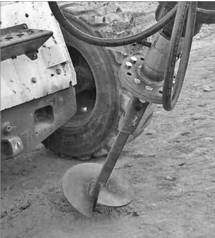
A skidsteer with a torque motor attachment is used to install the Helical Ground Anchor at the prescribed angle and depth for bracing.
