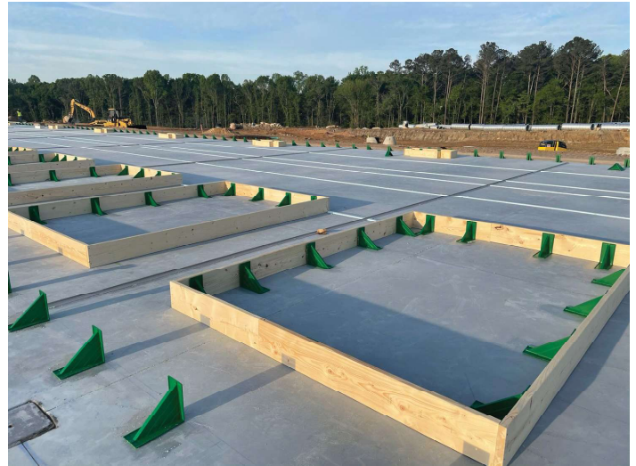
Construction Adhesive Edge Form Bracket Installation
