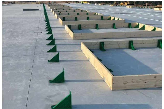
Construction Adhesive Edge Form Bracket Installation
