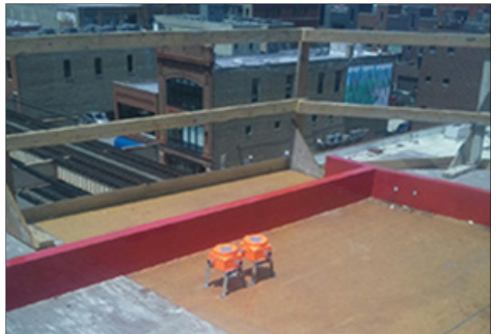
Ends can be overlapped or Slab Edge Corners and Fillers can be supplied to match the floor plan.
