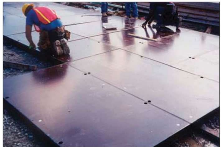
Long-lasting 3/4" birch plywood is the standard form face for Quick-Form panels.
