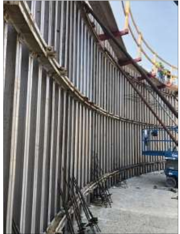
Radius forms can be reconfigured to match changing radius and wall dimensions.
