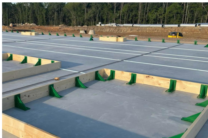
All Weather Adhesive used for Edge Form Bracket and chamfer installation
