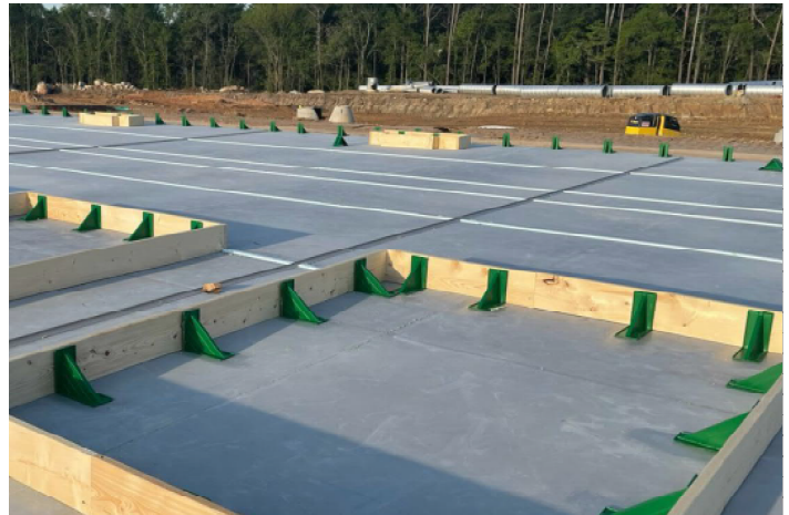
All Weather Adhesive used for Edge Form Bracket and chamfer installation
