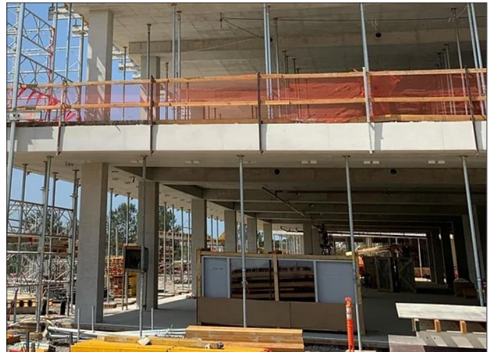
Post Shores can be used for supporting plywood decks or reshoring existing structures.
